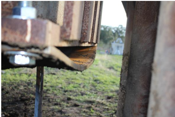
Figure 16: Post-test photograph with corner bolt still holding but showing where three bolts along the edge had failed (with the opposite corner still holding), thus allowing the hull edge to permanently deform.
